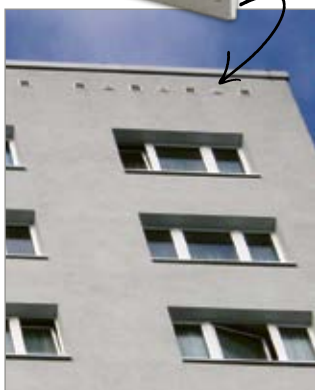
▲ Installation example for several Swift Cavity Panels
