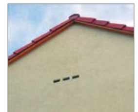
▲ three elements of 2FR installed flush with the façade
