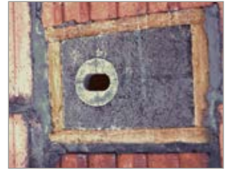
▲ on-site insulation to avoid thermal bridges
