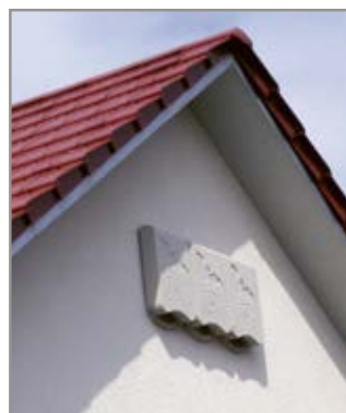
▲ 3 x 1WQ roosts installed in a group
